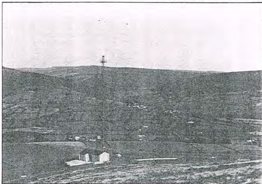
Shatton Edge. The 'slimline' tower was originally developed for use in the Peak District National Park. The 'trough' receiving aerials are just above the special stone building. The cantilevered cylinder contains a 'cardioid' transmitting aerial.
